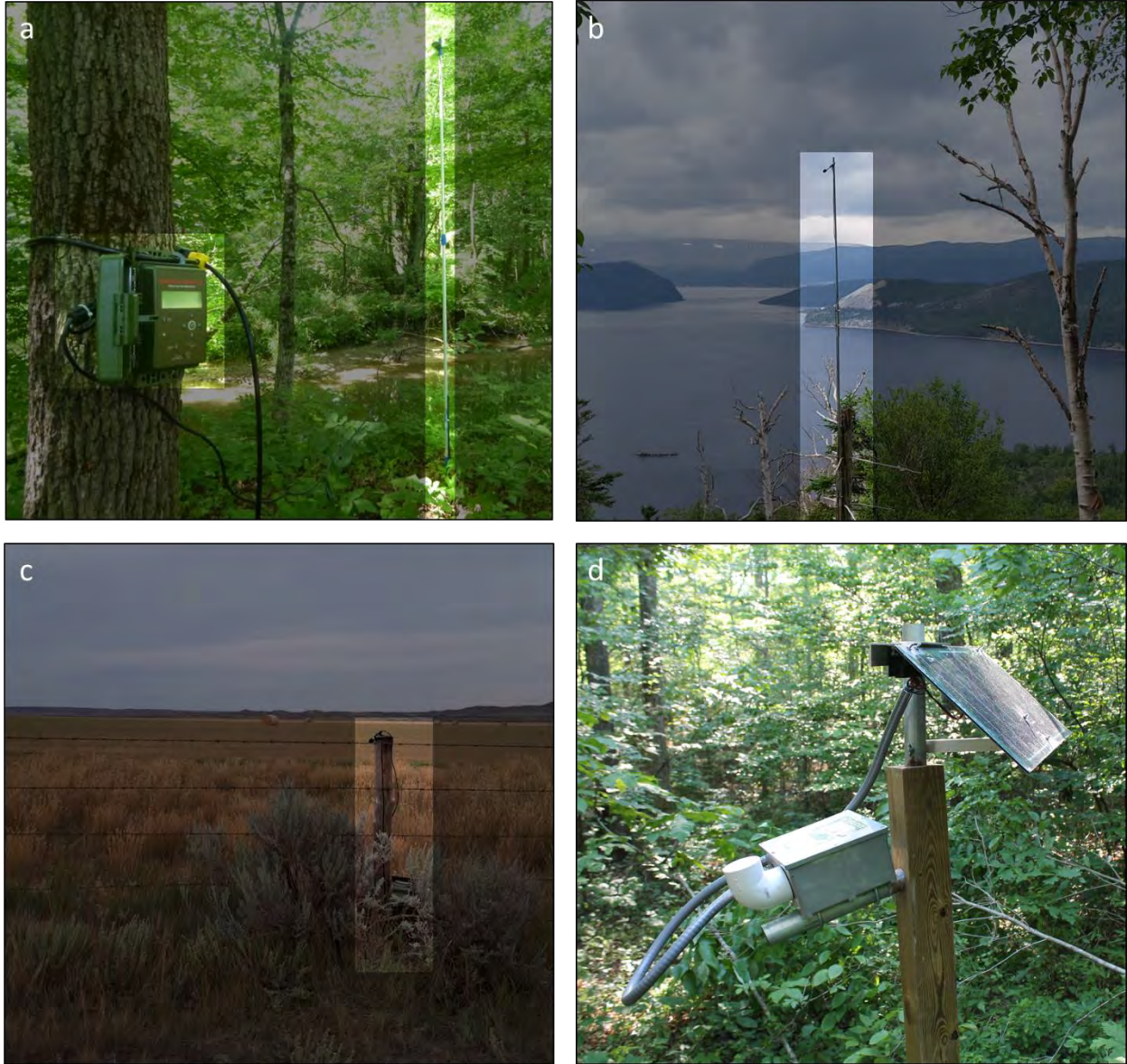
Figure 3-3. Examples of bat detector deployment. Actual bat detector deployments demonstrating a small sample of the variety of deployment techniques. Bat detectors, microphones, and deployment devices are highlighted in lighter shaded areas of the images. Image (a) shows a bat detector attached to a tree with a locking cable and microphone elevated on an extensible pole; sampling area is sub-canopy and comprises open forest understory and the small stream seen in the background © Alexander Silvis. Image (b) shows a microphone elevated on a pole attached to a snag; sampling area is above canopy © Darrian Washinger. Image (c) shows a microphone deployed on a fence post with the bat detector at the bottom of the post © Erin Swerdfeger. Image (d) shows a long-term acoustical monitoring station comprising a directional microphone, detector, and power supply in weatherproof housing accompanied by a solar panel; this system includes remote data upload using cellular technology © Alexander Silvis.
