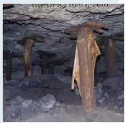
Stull buckling under increasing pressure of the ceiling settling over time.
