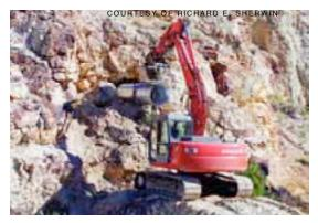
Culverts can be used to stabilize the entrance to a mine and provide a solid substrate for the attachment of a bat gate.
