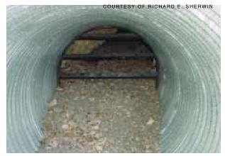
Protective closures (e.g., bat gates, fencing, etc.) must be routinely monitored to ensure their structural integrity and that they function as designed. This culvert with a bat gate has been blocked by erosion and requires maintenance.
